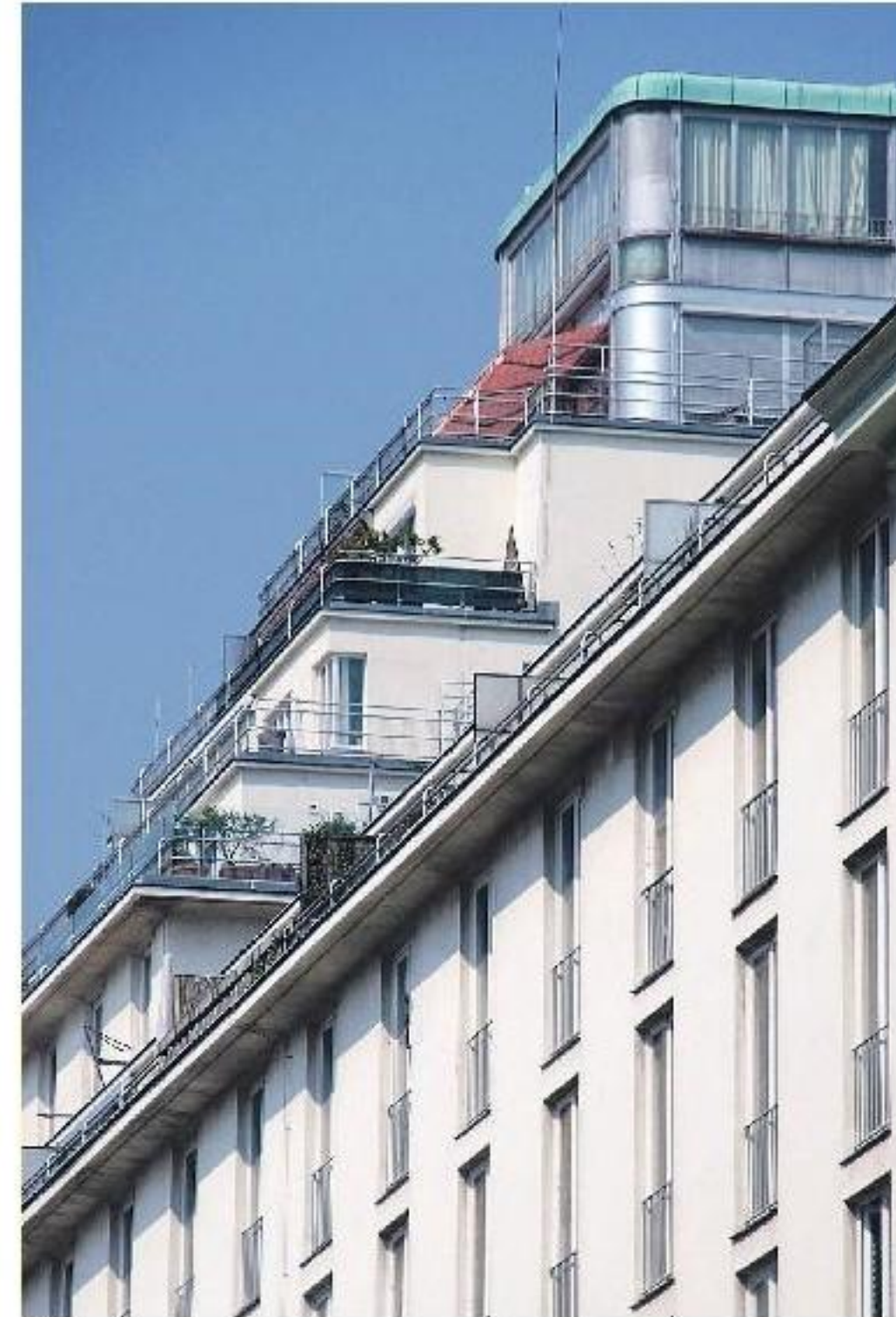
The stepped roof of the Hochhaus is to mask the building's height Photo: Duncan J.D. Smith
